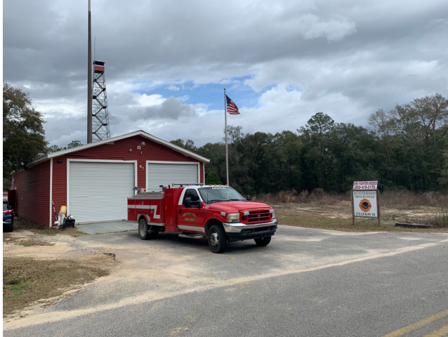
Station 91 67 Fire Department Avenue (Headquarters)
